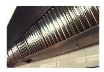
A properly designed, installed and functional ventilation system is critical for building fire safety. It is required to remove smoke odors and grease laden vapors from the cooking area to the exterior of the building. For this reason, it is imperative that the system is operating during all cooking periods and should operate for a minimum of 15 minutes after cooking has stopped. Below are recommendations for optimal ventilation system performance.
