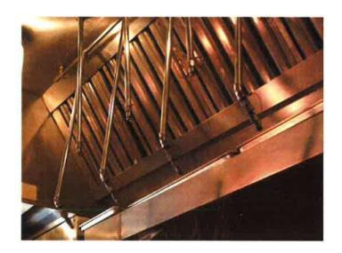
Older suppression systems use dry powder as a suppression agent, which will not create a foam barrier with vegetable oil appliances and could lead to re-ignition. For this reason, older dry powder systems need to be replaced with a UL-300 compliant wet type system.
